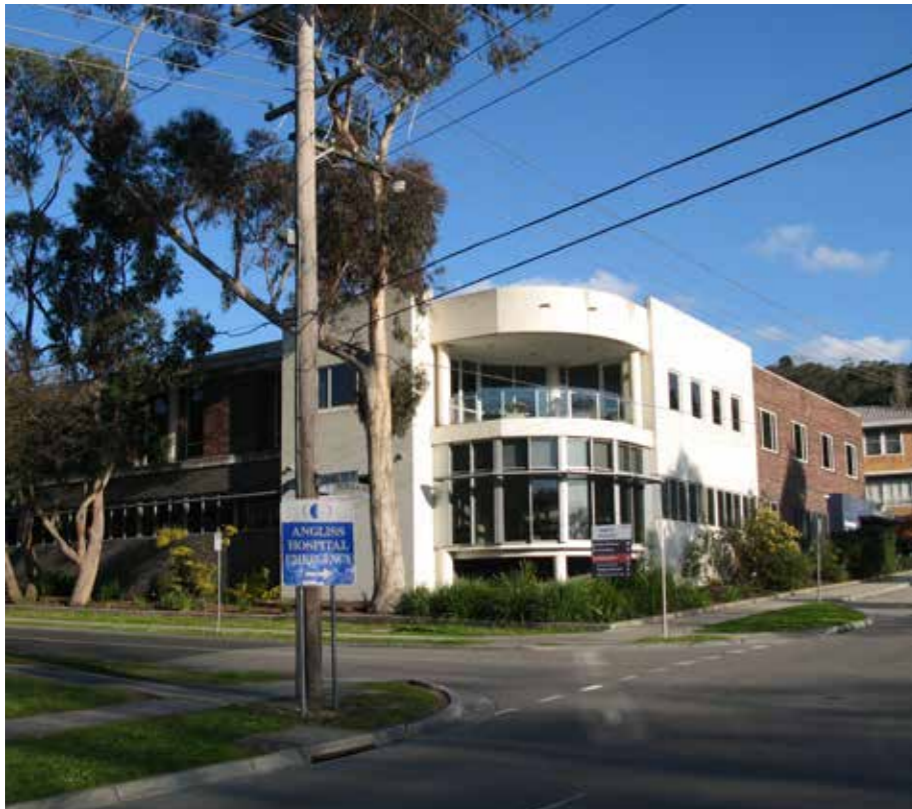
The Angliss Public Hospital and supporting health uses
