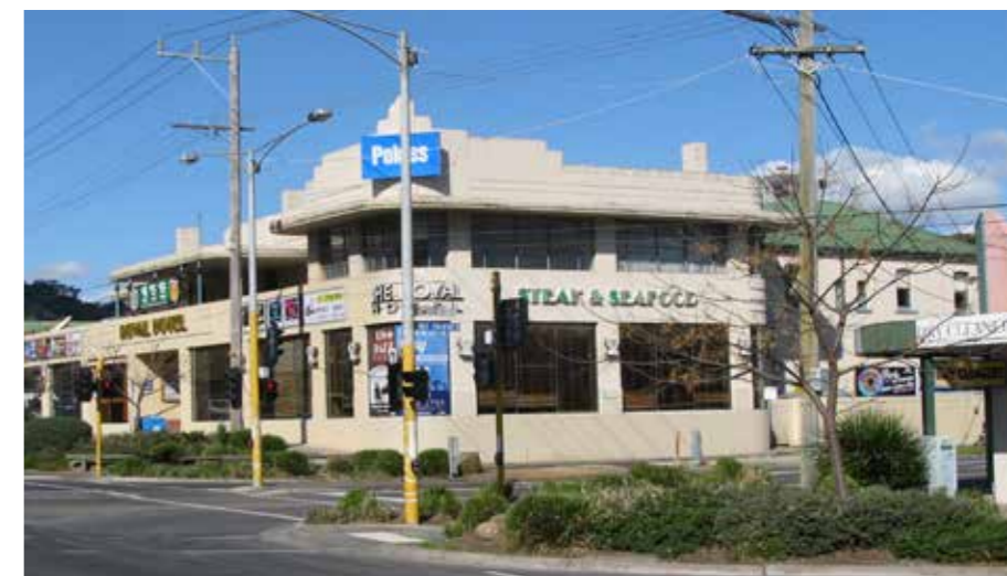
The Royal Hotel is a land mark building in Upper Ferntree Gully
