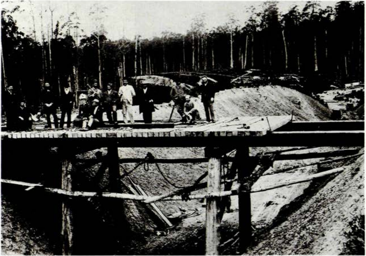
Railway construction near Korumburra
