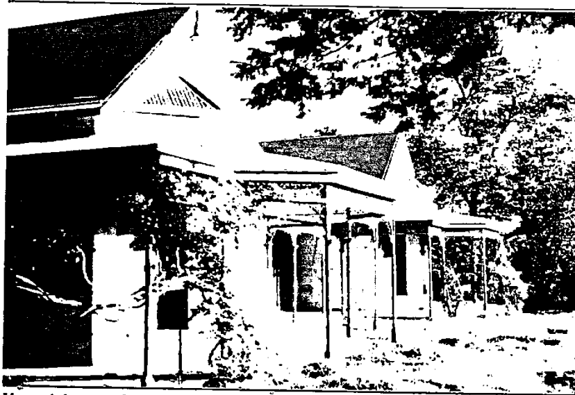
Verandah area of Stamford Park during early restoration work in 1990.
