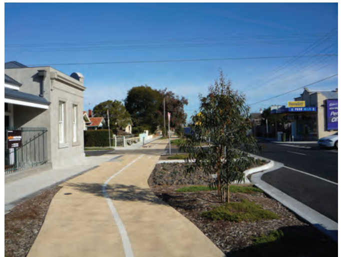
O'Hea Street, Coburg showing an off-road shared path, footpath and rain garden in mulched nature strip
