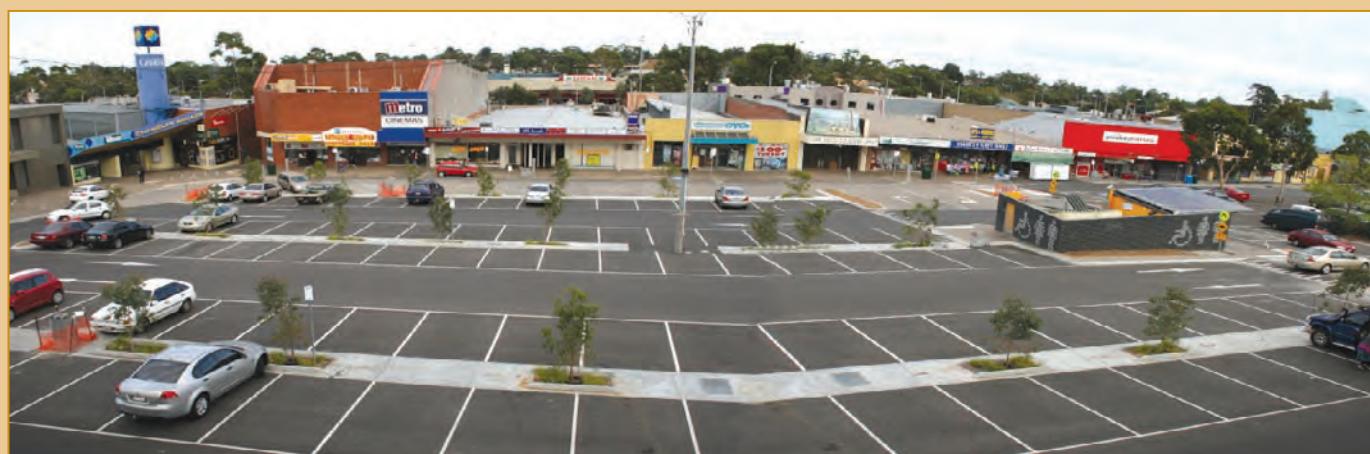
Boronia car park was retrofitted with water sensitive urban design and new street trees.
