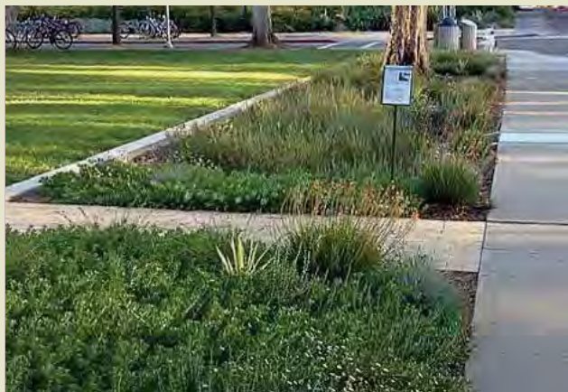
Sunken planted water detention strips lining the road.
