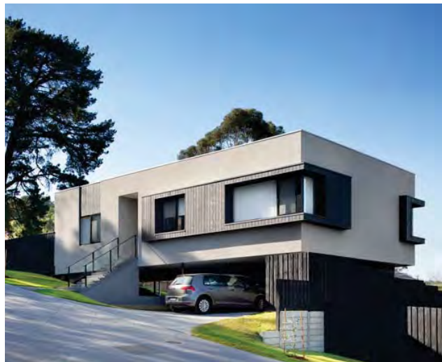
HighWood, completed in 2017.
