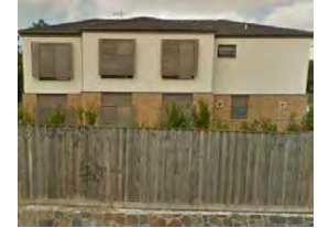
No. 184 Dorset Road UNIT 1 Double-storey brick & wood veneer with pitched roof
