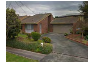
No. 184 Dorset Road UNIT 2 Single-storey brick veneer with pitched roof
