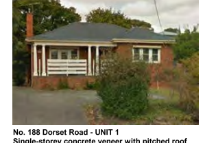
No. 188 Dorset Road - UNIT 1 Single-storey concrete veneer with pitched roof
