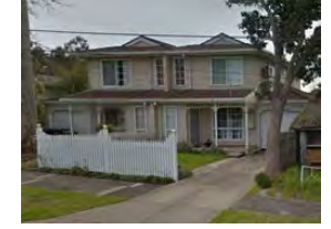
No. 182 Dorset Road - UNIT 2 Double-storey wood veneer with pitched roof
