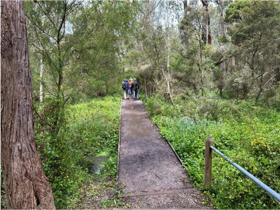
Pedestrian Crossing of Forest Road Drain
