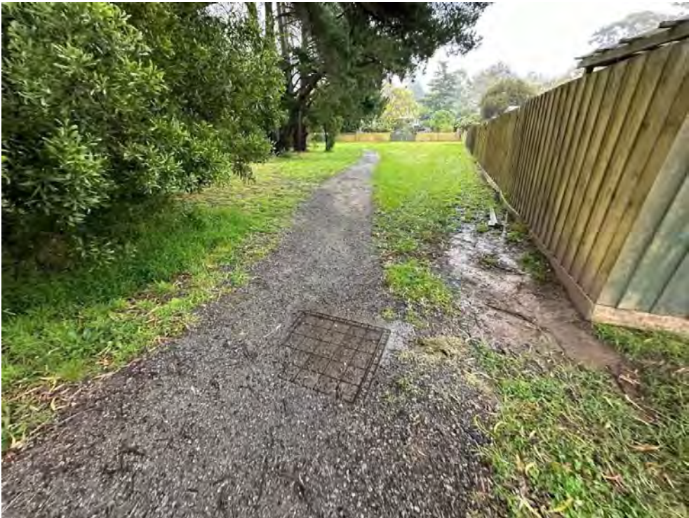
Walking Track at Rear of Daffodil Road Properties looking West
