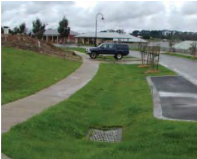
Figure 3.7: Grassed Swale – Source: CSIRO (2005)
