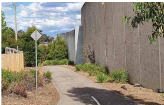
The noise barrier should be located within the EastLink reserve on the eastern side of the EastLink Trail.
