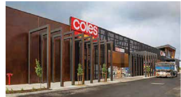
Where practical, integrate loading and servicing areas into the design of the building.
