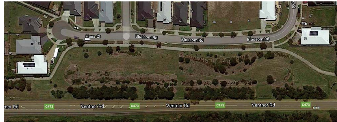
Example dry detention basin with rain garden cells in Cowes, Victoria.
