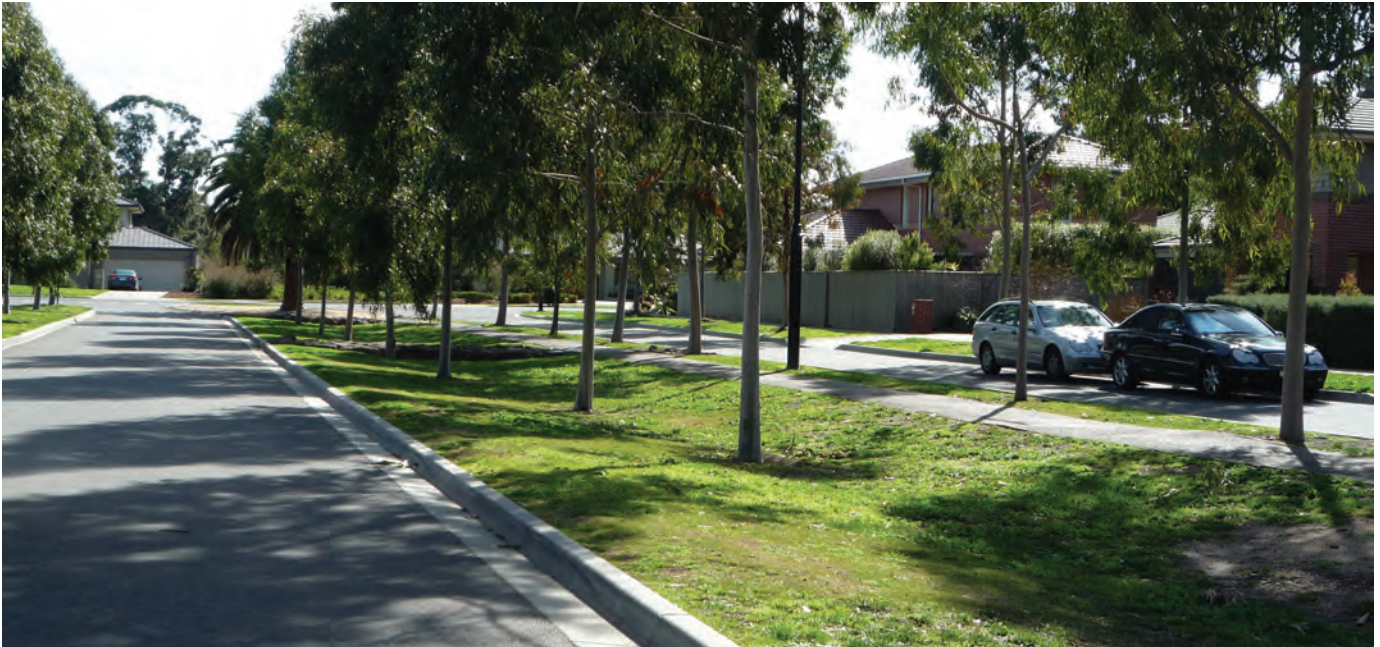
A street with a central swale to capture and clean the storm water from the carriageway, Springthorpe, Macleod
