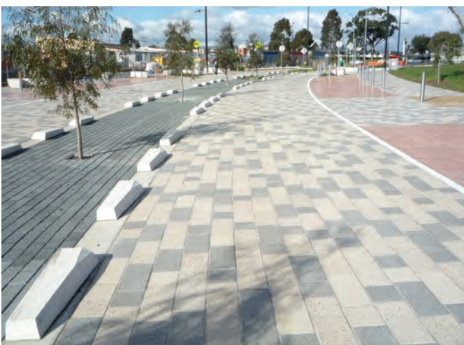
Shared street, Main Street, Broadmeadows, showing various materials to decrease driver speed
