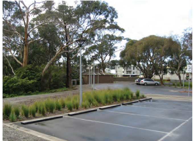
Water sensitive urban design treatment in a carpark
