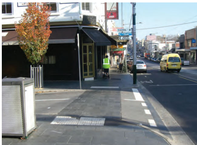
Crossing point, South Yarra showing the road raised to pedestrian level and paved in the foot path material, to prioritise pedestrians
