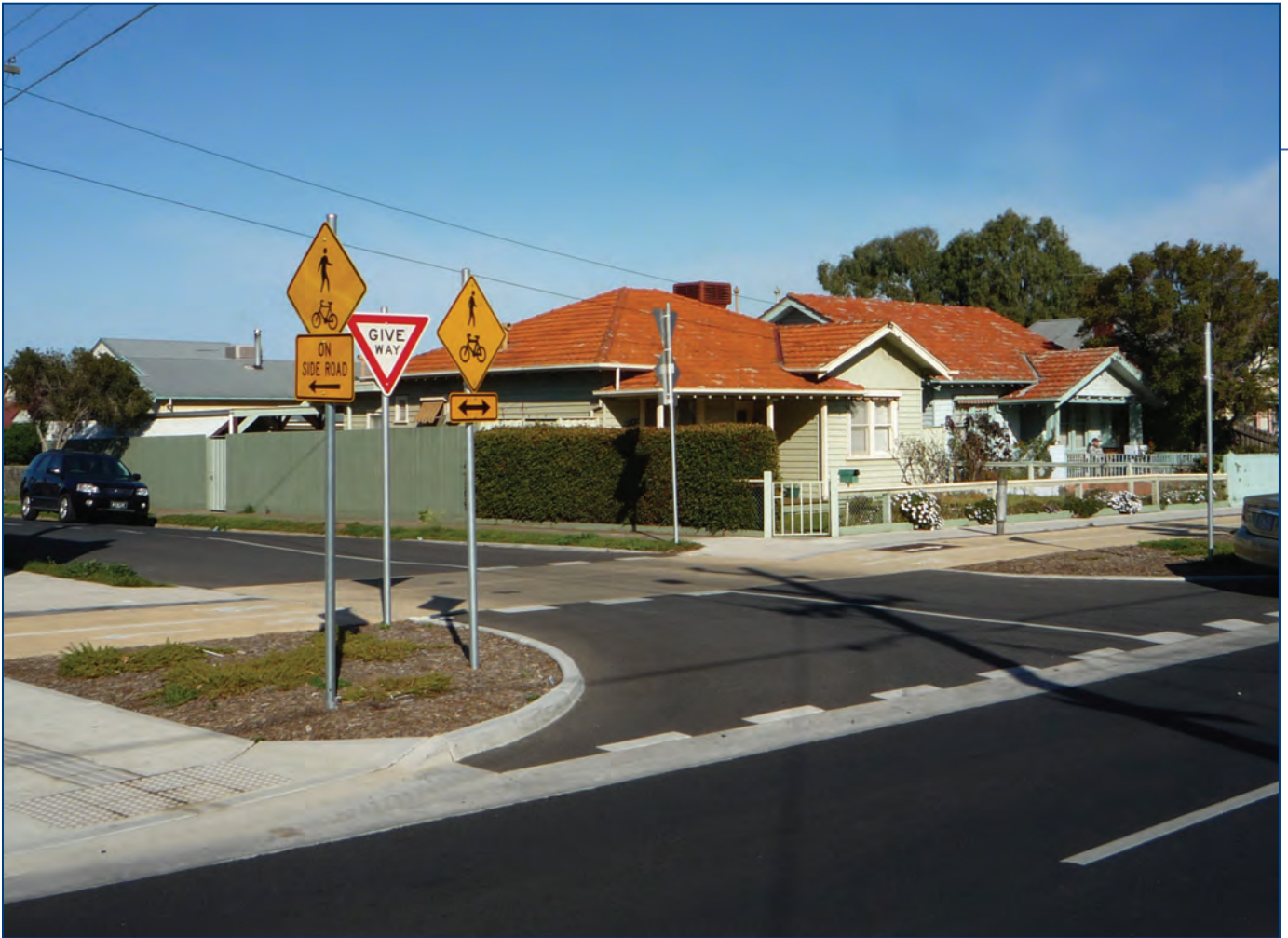
O'hay Street, Coburg with an off-road shared path. Cars give way to pedestrians and cyclists at crossing points
