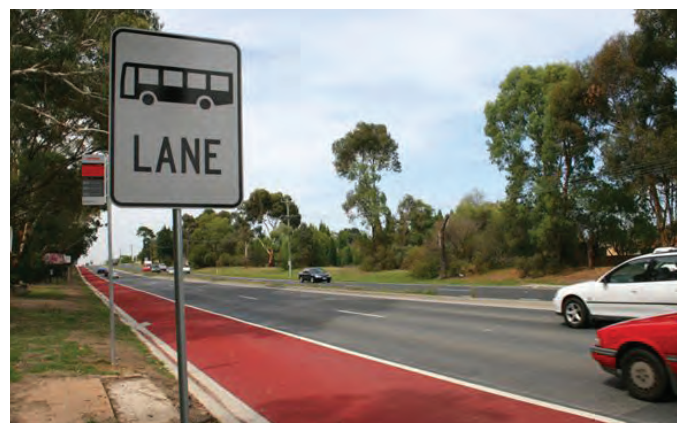
Bus lane on Stud Road
