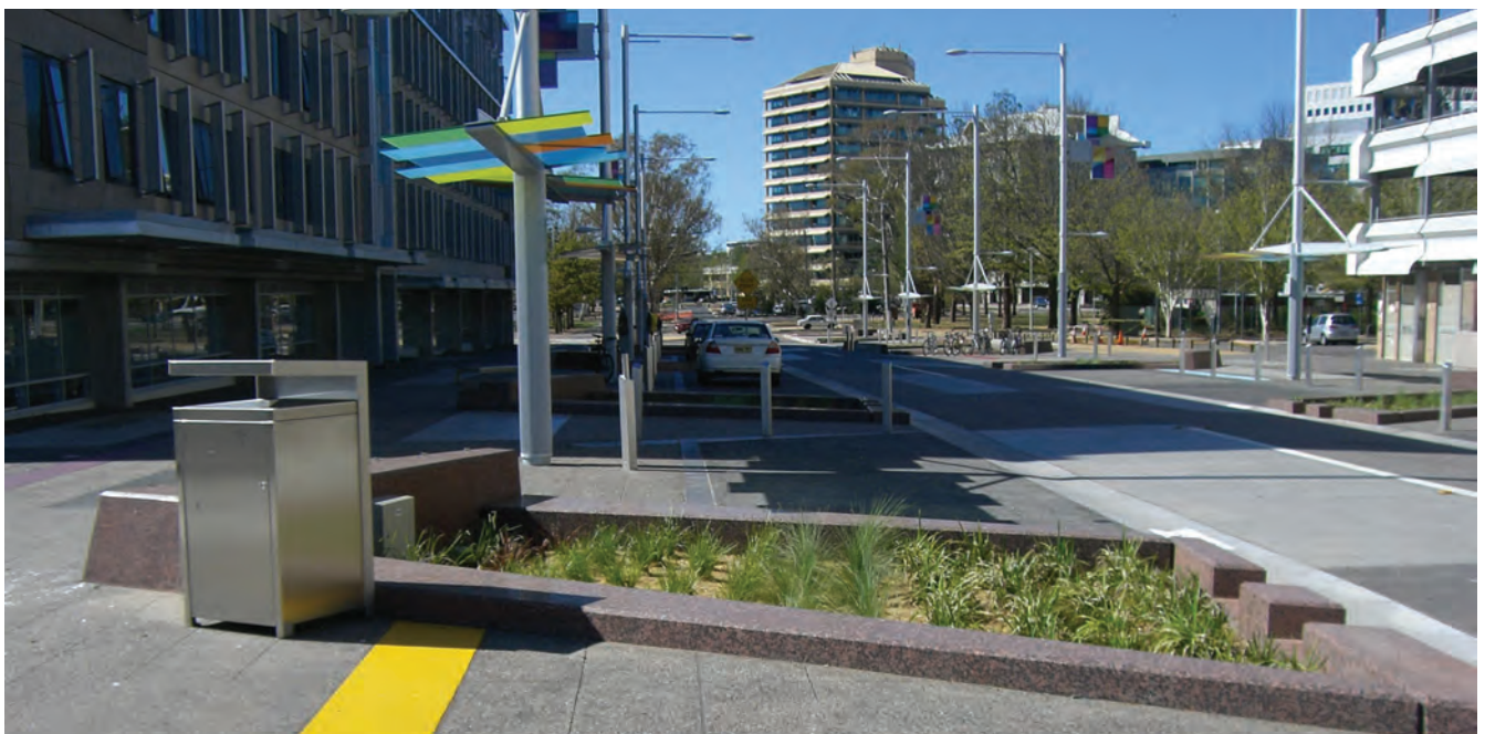
Shared space in Canberra with water sensitive urban design treatment gardens
