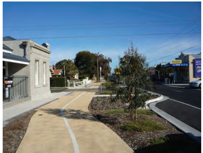
O'Hea Street, Coburg showing an off-road shared path, footpath and rain garden in mulched nature strip
