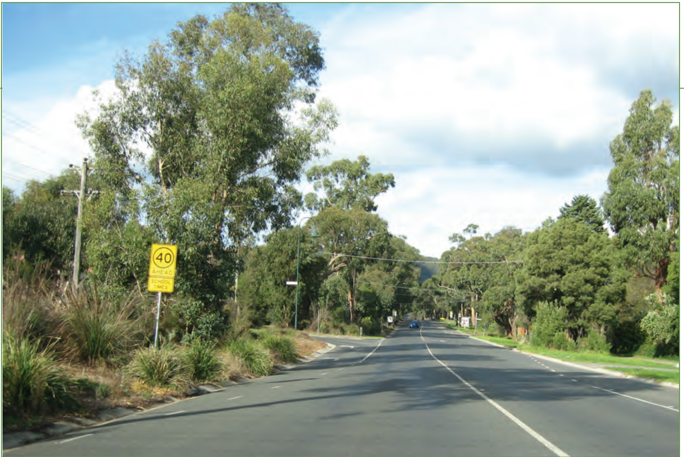
Mountain Highway, Boronia showing a roadway Site of Biological Significance
