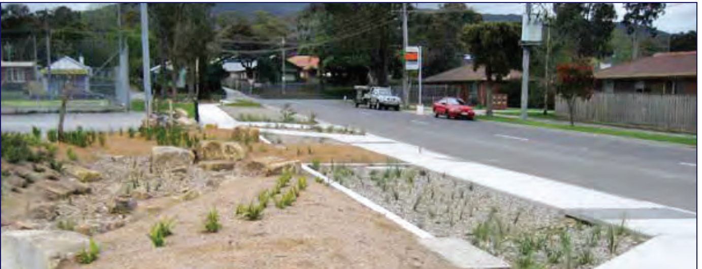
Recent street projects in Knox have used water sensitive urban design to improve water quality in Knox's waterways. Photograph in Boronia
