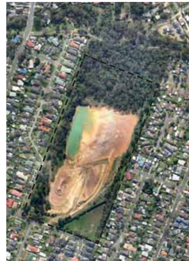
Figure 11 Site in Sept 2013
