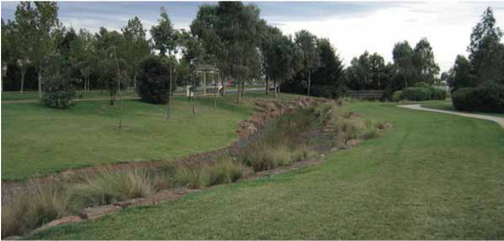
Figure 12 – Example of the vegetated swale to be created adjacent to the Bushland Reserve (Urbis, 2021).
