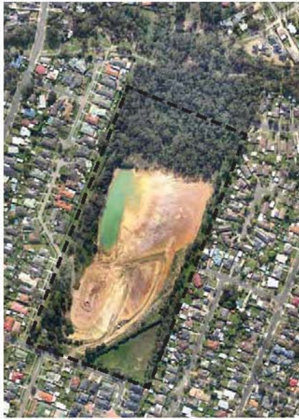
Figure 3 Site in Sept 2013
