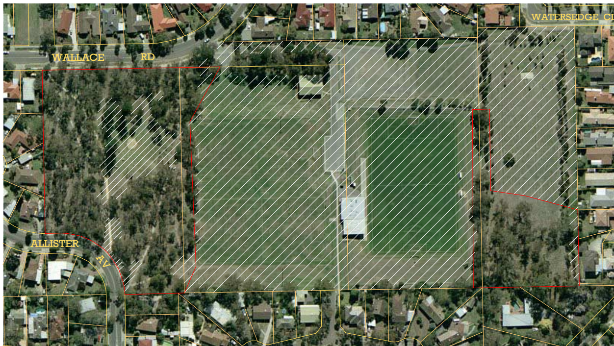
Aerial photograph taken April 2003
