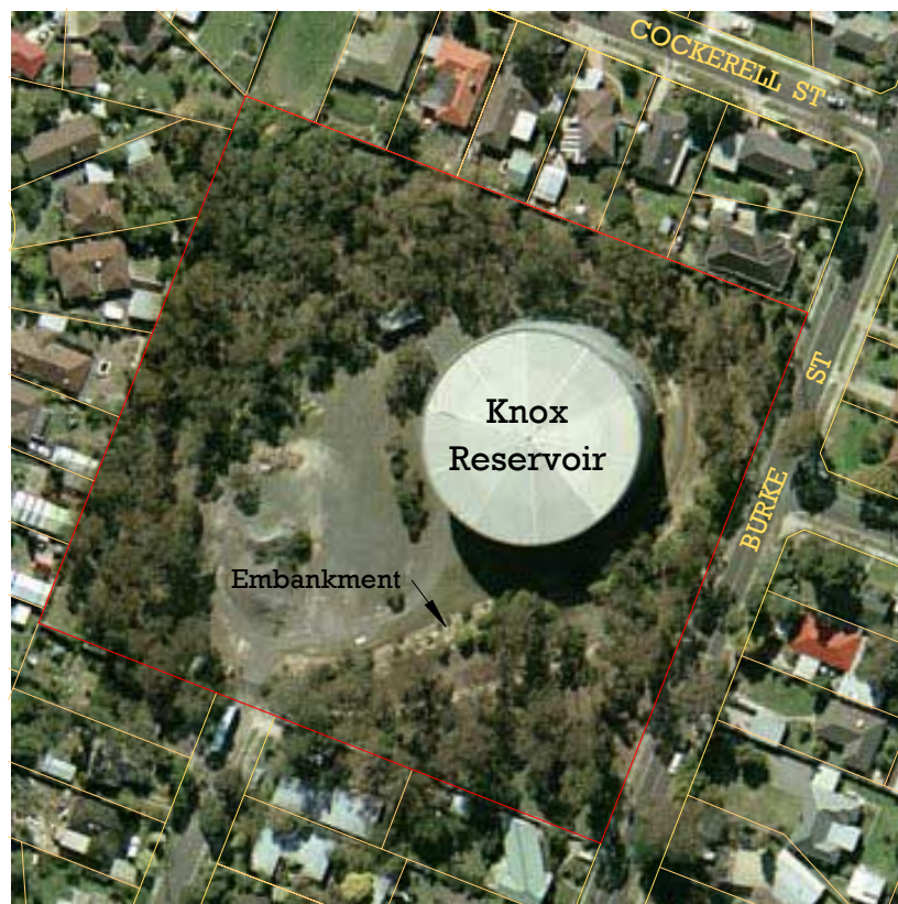
Aerial photograph taken April 2003
