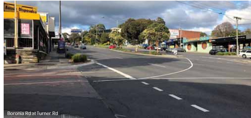
Boronia Rd at Turner Rd
