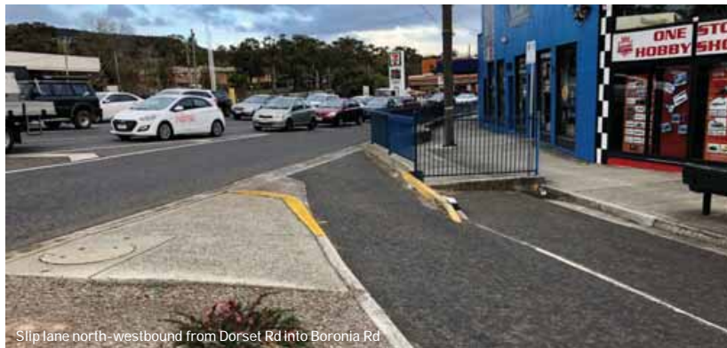
Slip lane north-westbound from Dorset Rd into Boronia Rd
