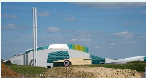
Ardley Energy Recovery Facility, UK
