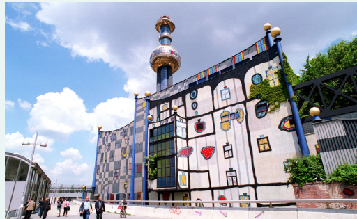
Spittelau Waste to Energy Facility, Austria
