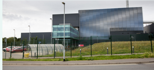
Suffolk Energy From Waste Facility, UK
