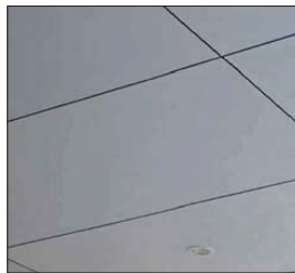
FC-1 Expressed Joint Sheet Cladding Soffit
