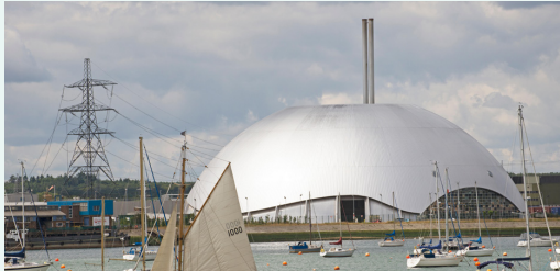
Marchwood Energy Recovery Facility, UK
