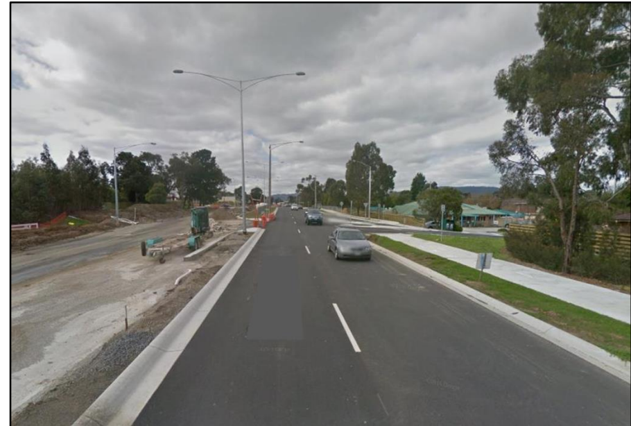
Figure 3-5 High Street Road Improvement Works (September 2015)
