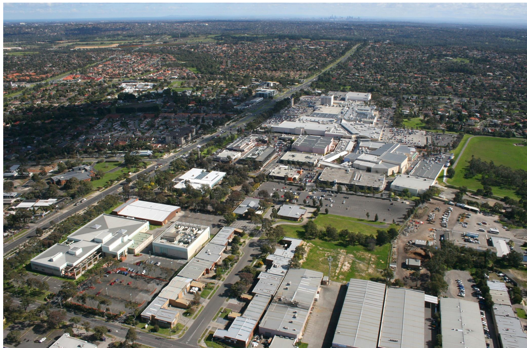
Figure 10 Aerial photo showing Knox Central's built form
