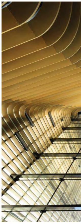
Sir Louis Matheson Library - Window Wall Facade - Aluminium fins
