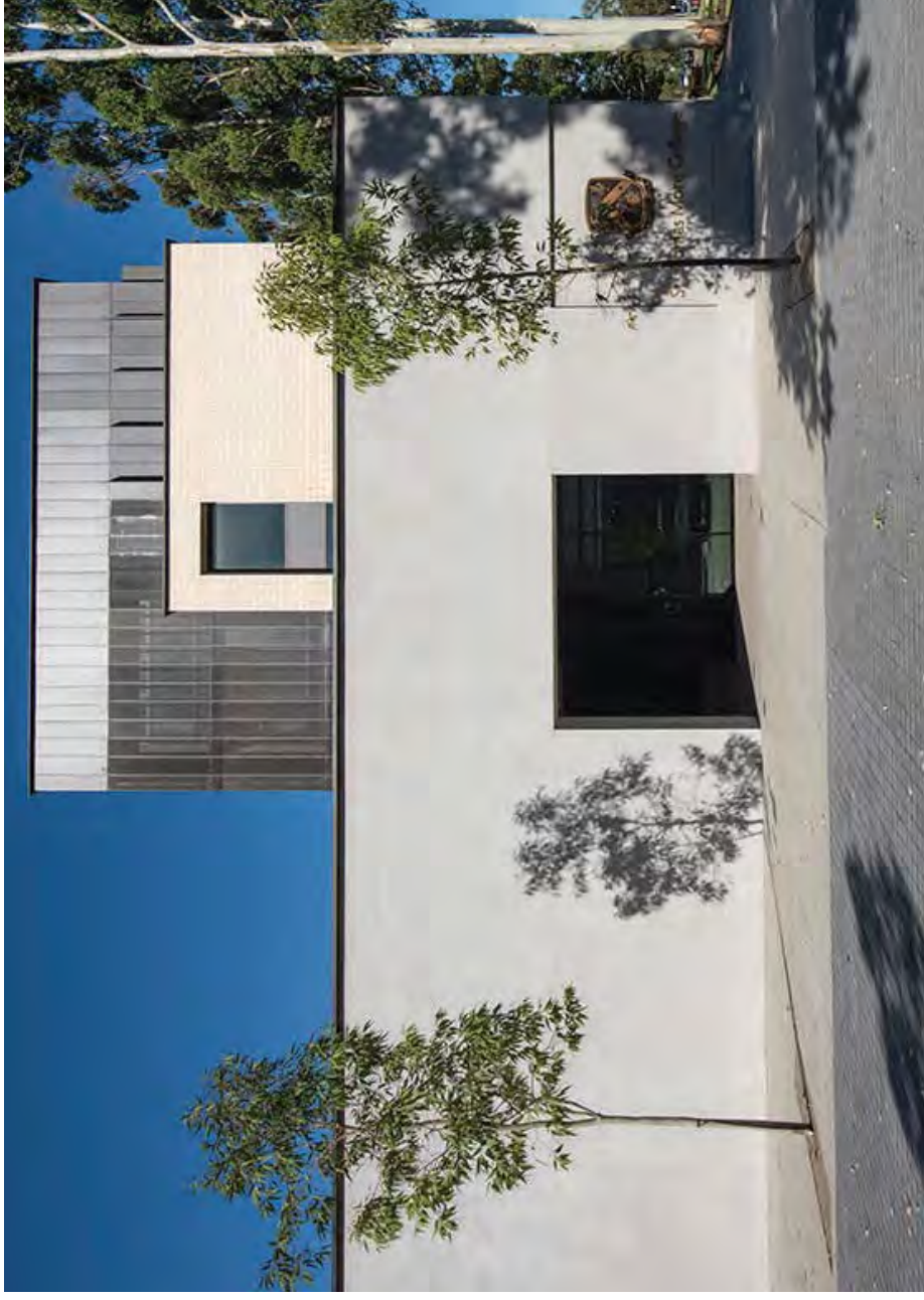
St Thomas More College - Perforated sheet screen -Pre Cast Concrete
