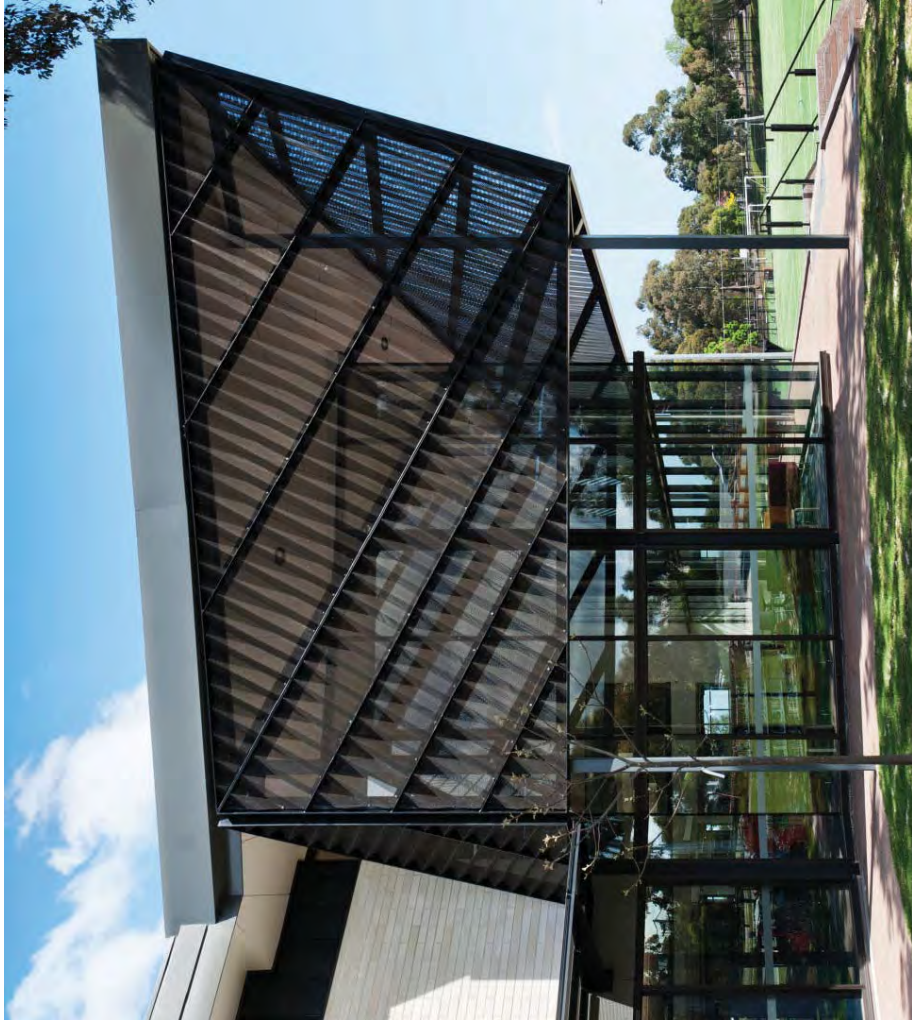
Presbyterian Ladies College - Folded perforated sheet screen - Clear glass, window wall facade
