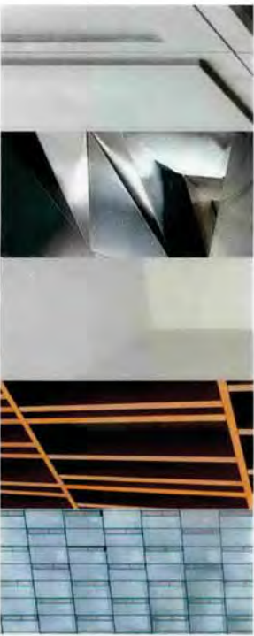
GLA 01 Light Colour Glass Facade PCT 01 Powder Coated Bronze Fin SOFF 01 Painted Soffit PCT 02 Powder Coated Metal CONC 01 Precast Concrete
