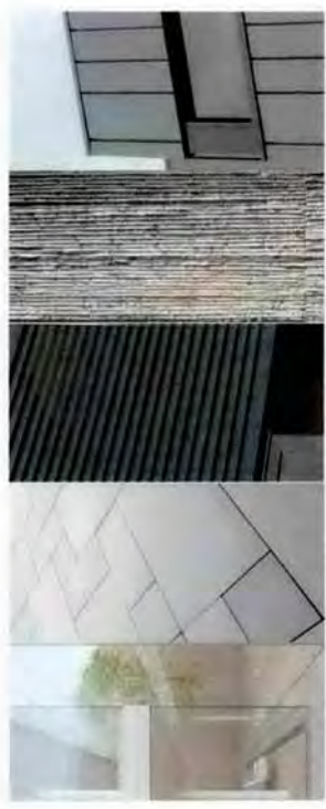
GLA 02 Shopfront Glass PAV 02 Concrete Paving LVR 02 Charcoal Colour Aluminium Louver CONC 02 Textured Precast Concrete ALUM 01 ALUMINIUM CLADDING
