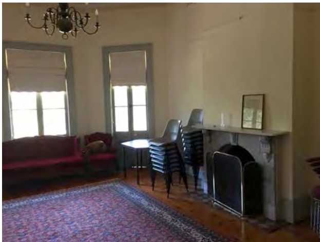
View of front room on left with canted bay. Note marble fireplace with original cream and red tiled hearth (a matching fireplace is in the roof directly opposite)
