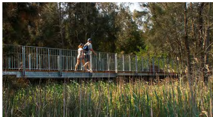
Bridge over sensitive vegetation
