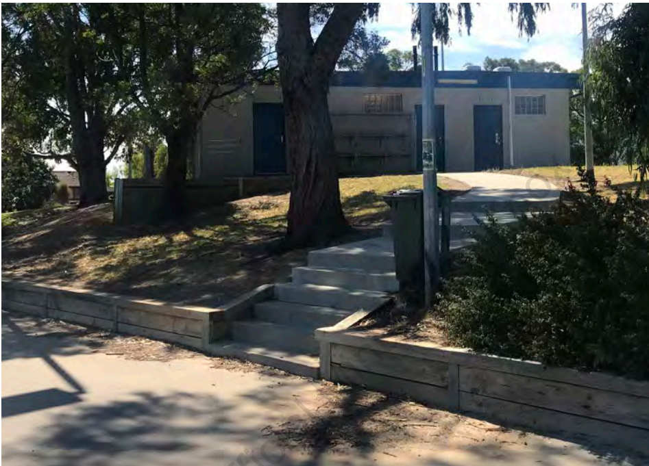
Steps and path leading to toilet/changing facilities, located within the football/cricket pavilion.
