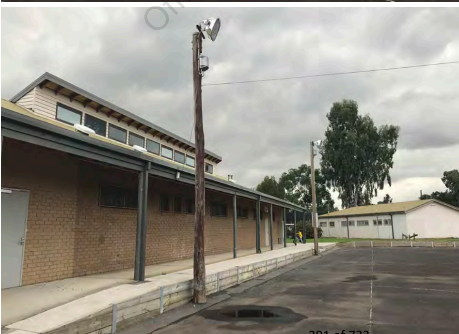
The cricket/soccer pavilion abuts the south-western edge of the courts.
