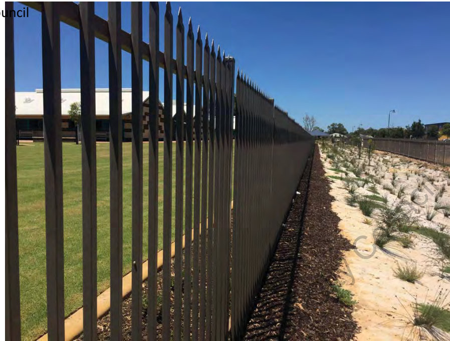
FENCE TYPE 1- PALISADE STYLE
