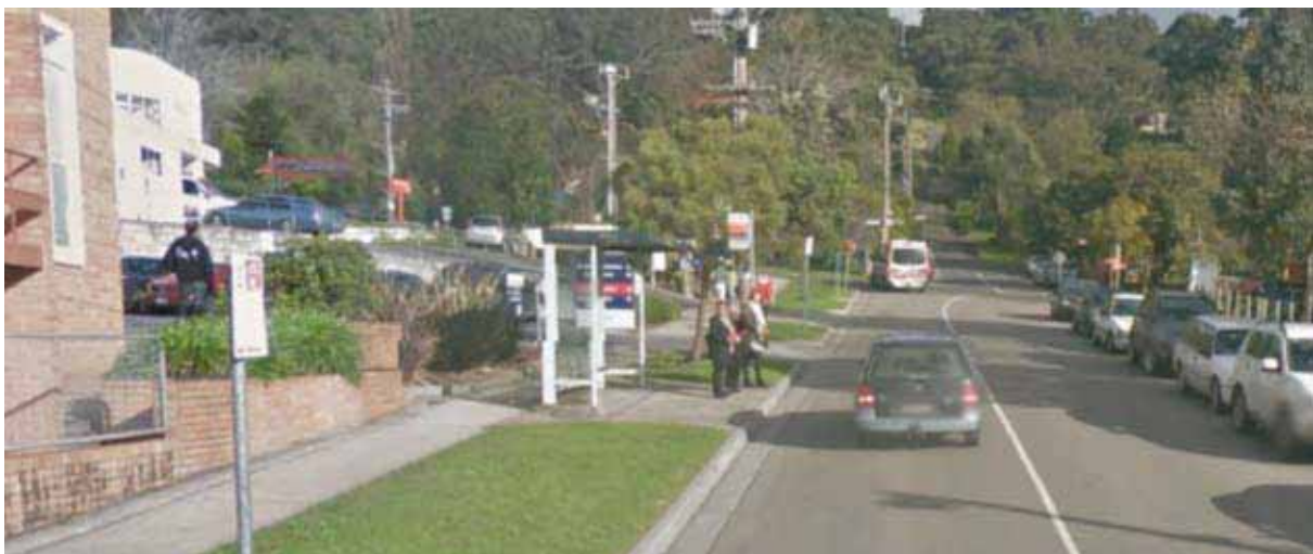
Figure 29: Route 732 Extension Bus Stop on Talaskia Road – outside Angliss Hospital
