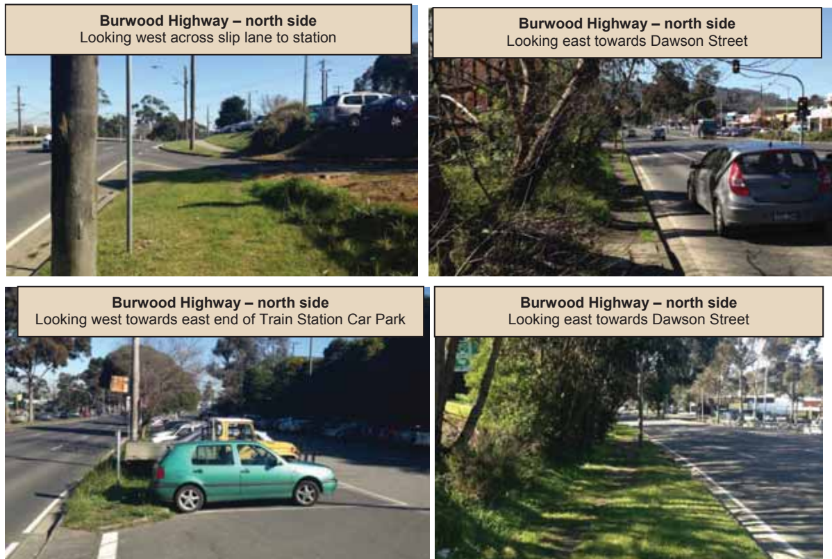
Figure 24: Lack of Footpath Facility on north side of Burwood Highway – adjacent to Train Station Car Park
