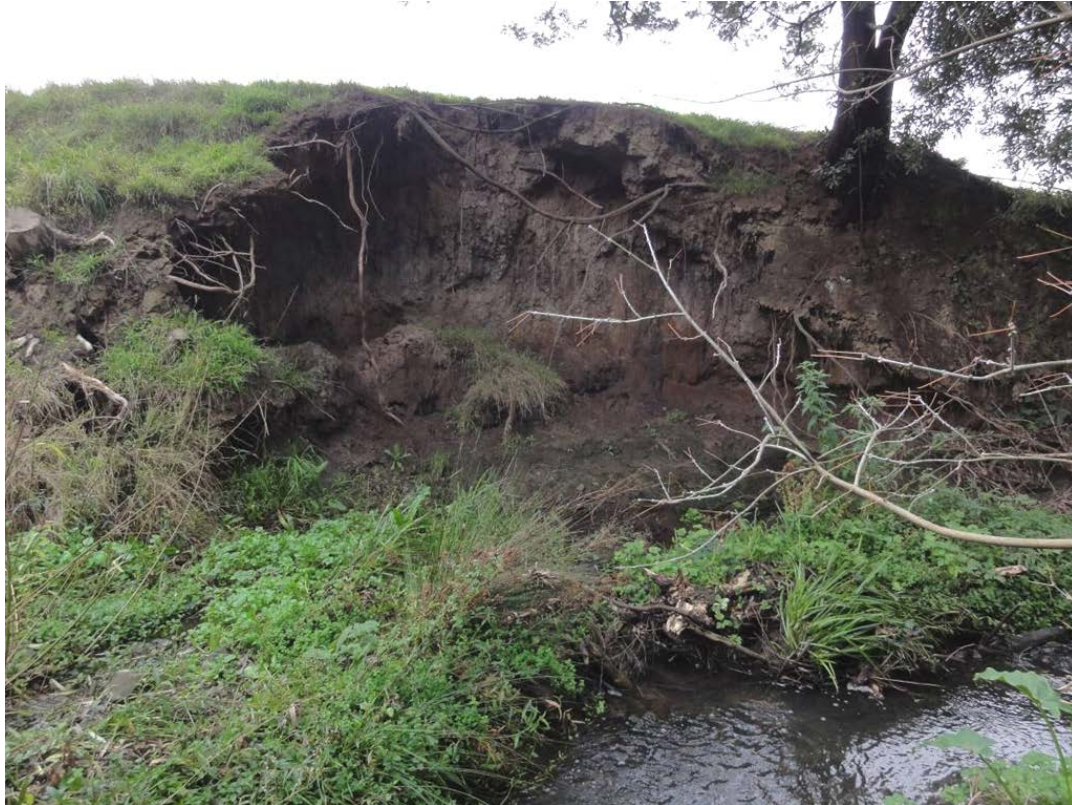
Figure 7. A dangerously undercut bank.
