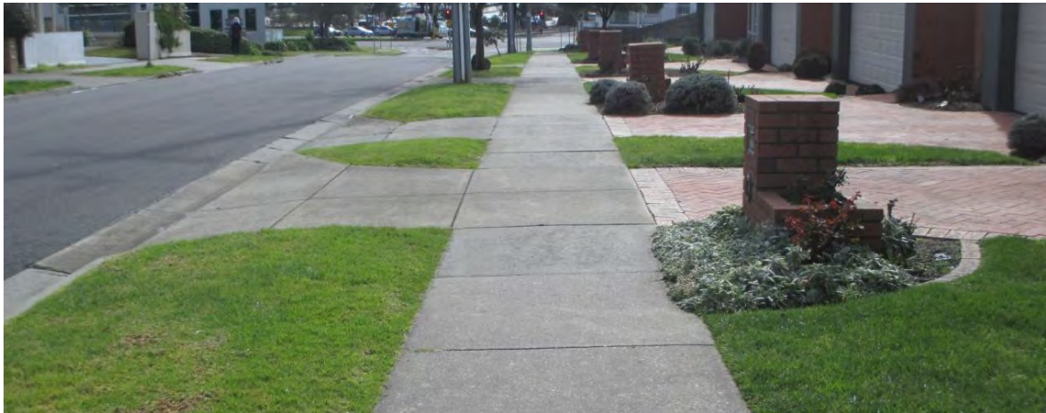
Figure 5 Typical footpath in a road reserve
